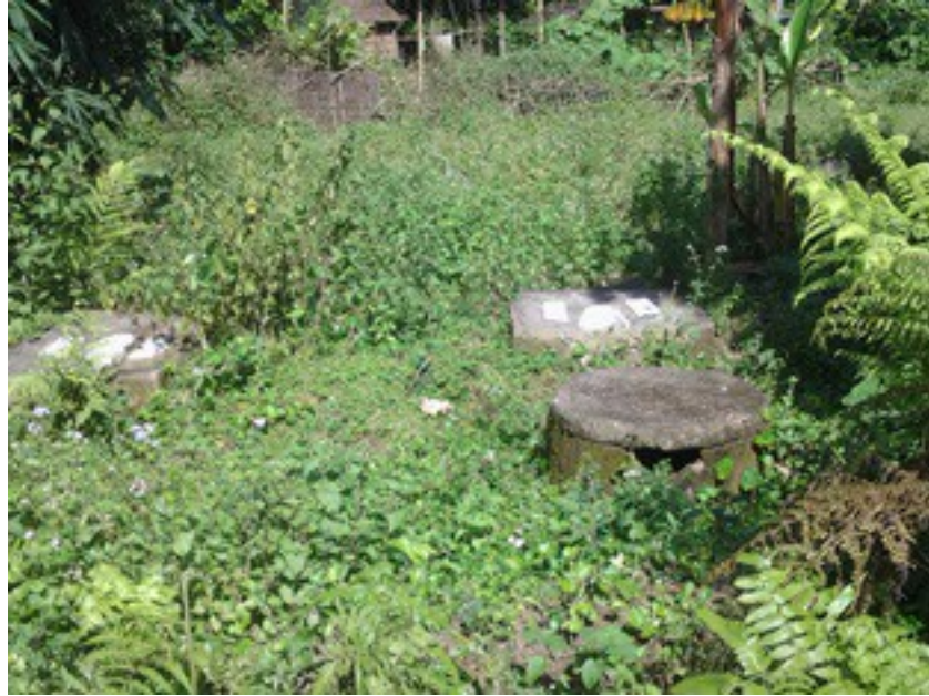
PHE constructed toilets remaining unused in Bhimpora village in Lakhimpur.
